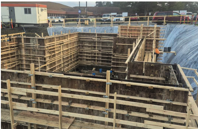
Construction progress at Jesse's House
